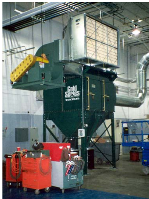
Cartridge collector equipped with safety monitoring filter bank.
